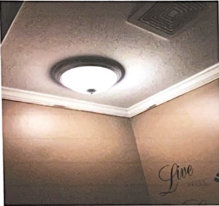
LIGHT FIXTURE IN BATHROOM REPLACED
