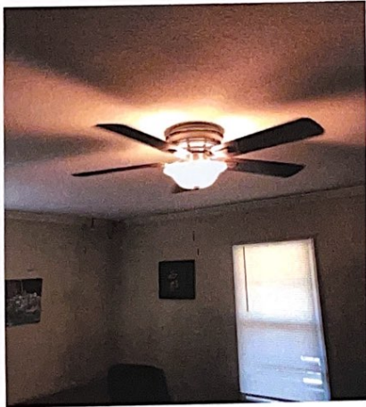
LIVING ROOM LIGHT FIXTURE REPLACED
